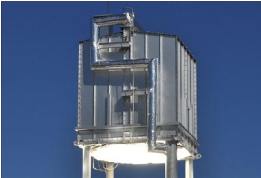
**Figure 91 Close up photograph of solar receiver utilising irradiated graphite [140].**
