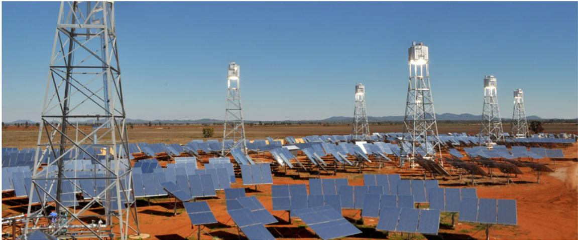
**Figure 90 Existing graphite storage/receivers developed by Graphite Energy. These graphite systems could be doped with some distributed immiscible fusible phase to create a Miscibility Gap Alloy system with higher energy density [140].**
